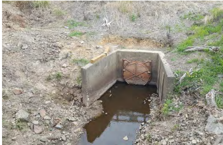
Figure 3: Outlet of gravity flow outlet pipe Okowhao Pump Station. Photo: Taroi Rawiri, Waahi Whaanui
