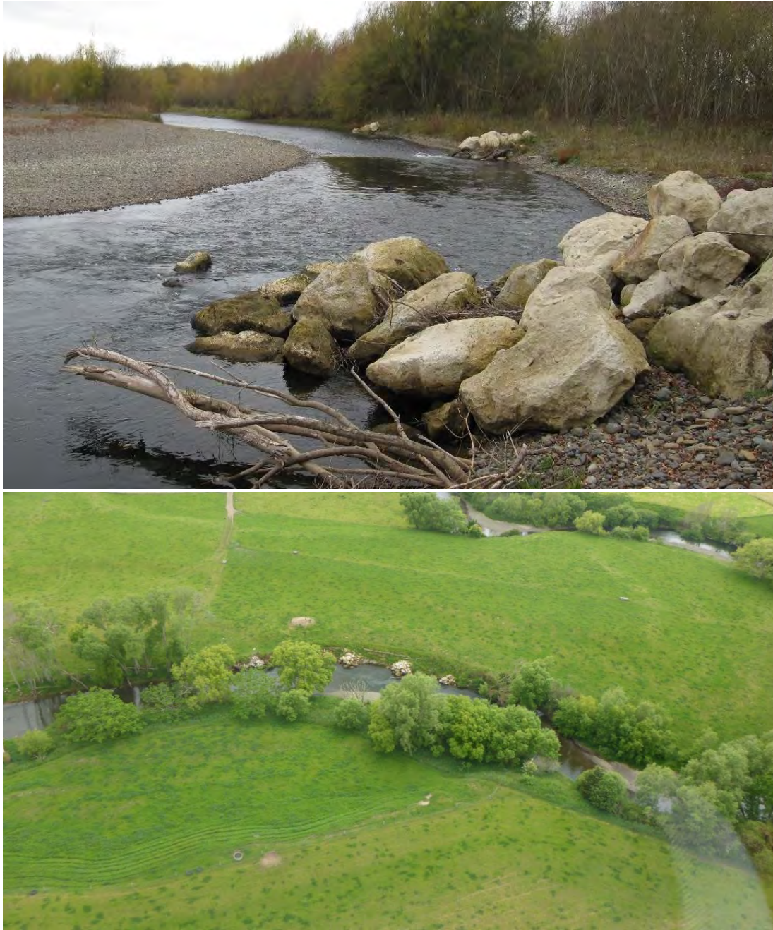
Examples of rock and vegetation erosion protection structures (as proposed as part of this project).
